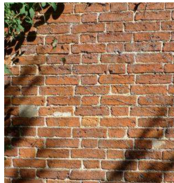
FIGURE 24: EXAMPLE OF TRADITIONAL LIME POINTING
