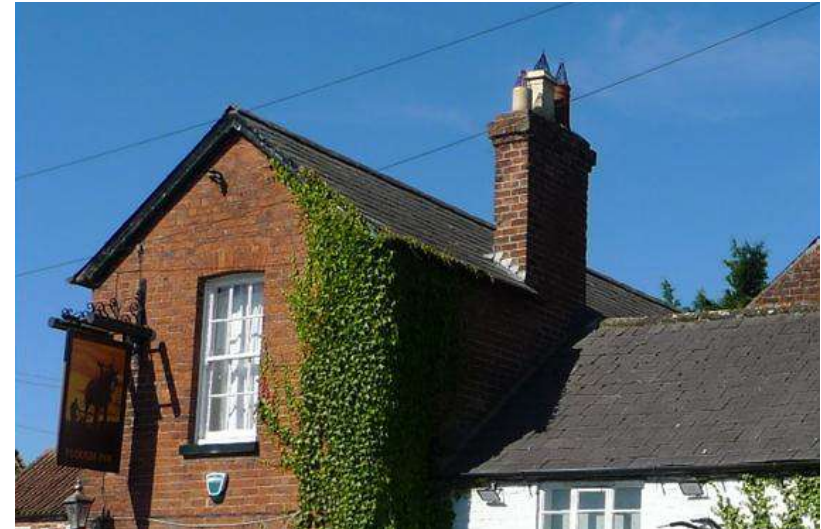
FIGURE 15: EXAMPLE OF A SLATE ROOF ON THE PLOUGH INN
