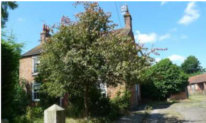
FIGURE 14: DETACHED HOUSES SET BACK FROM MAIN STREET WITH OPEN AREAS AROUND THE BUILDING AND FORMER FARM OUTBUILDING
