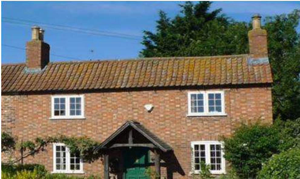
FIGURE 16: EXAMPLE OF A PANTILE ROOF
